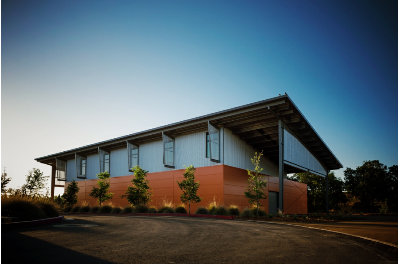
Vertical fins shade the windows of the JSWB. Photo: Courtesy Guttman & Blaevoet Consulting Engineers
